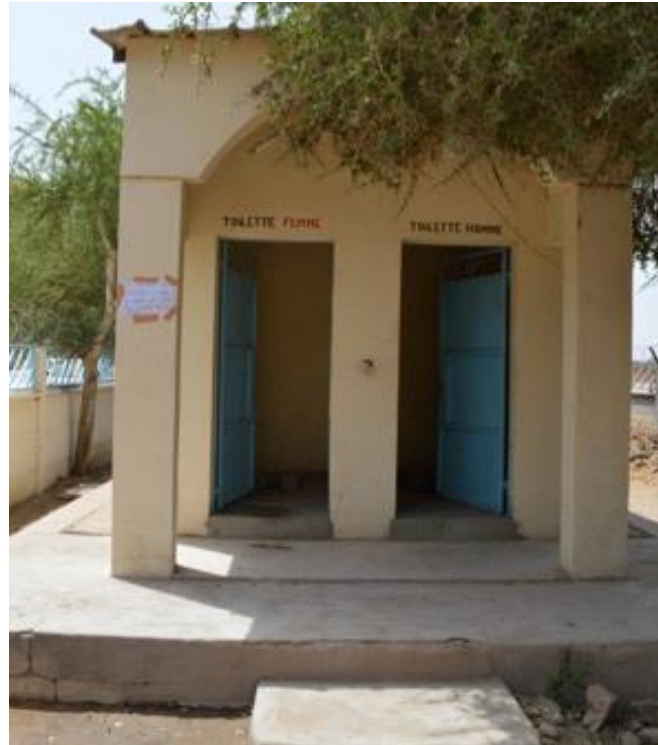
Clear signs demonstrating gender separation of latrines
